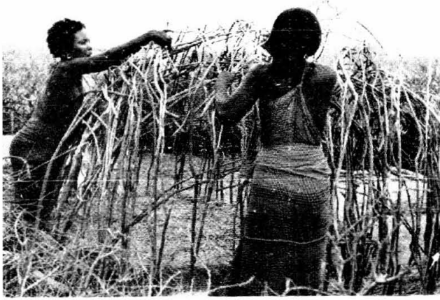
Building an akhal , the transportable thatched nomad hut.
