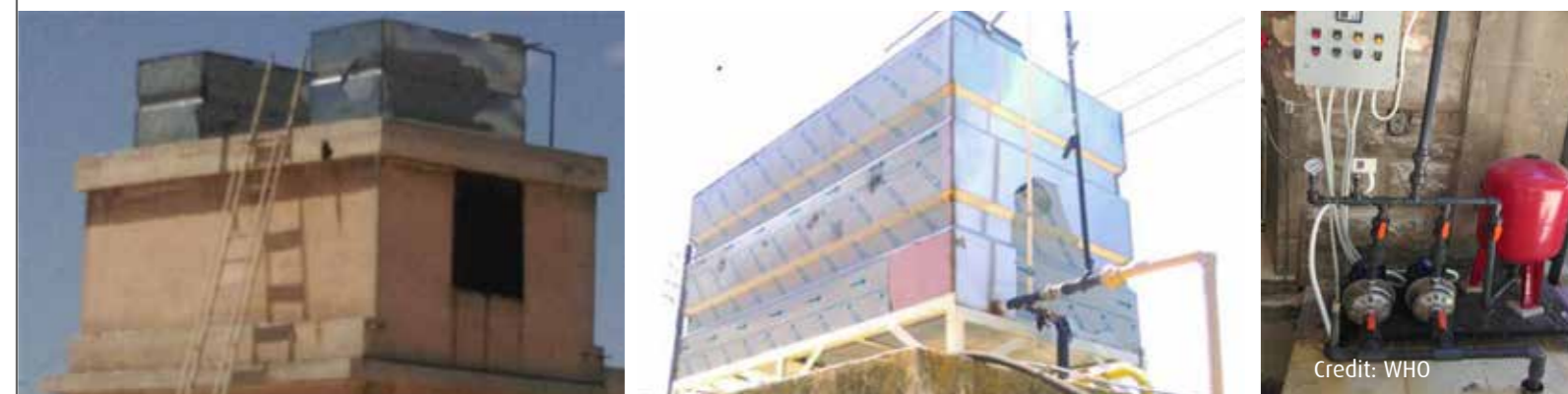
Stainless steel tanks installed in St. Louis Hospital in Aleppo, with new pumps to lift water to rooftop tanks.
